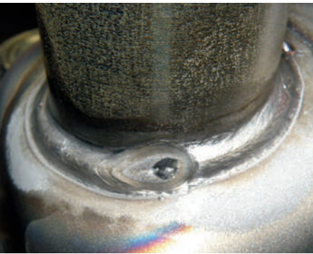
After water jetting
