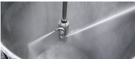
3rd gear – full pump power as typically employed for tank cleaning
