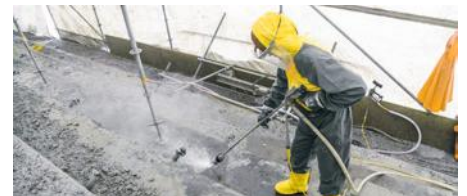
1st gear – low pump power for manual blasting gun work
